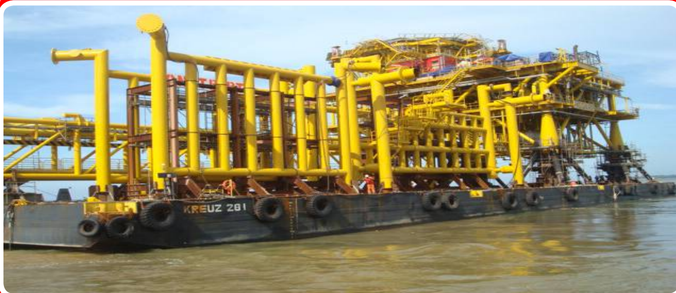
Loadout of Well Platform for Daman Development Project.
